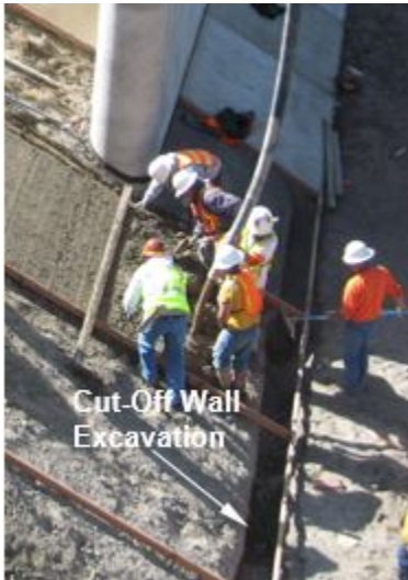
Figure 55: Slope paving cut-off wall excavation
