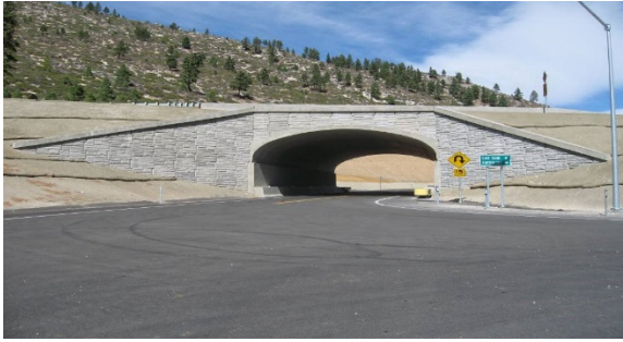
Figure 56: Typical MSE wall
