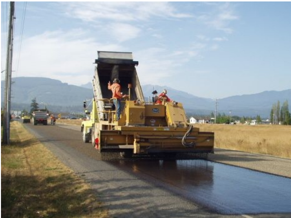
Figure 25: Chip spreader and hauling trucks
