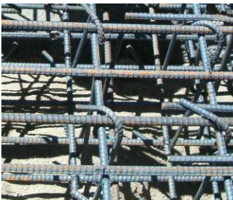
Figure 44: Reinforcing steel showing minor amounts of rust
