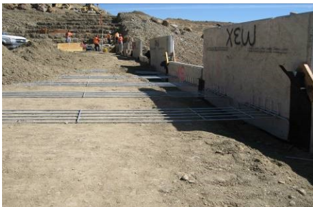
Figure 58: Soil reinforcement connected to MSE wall facing panel
