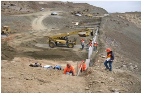
Figure 57: MSE wall installation
