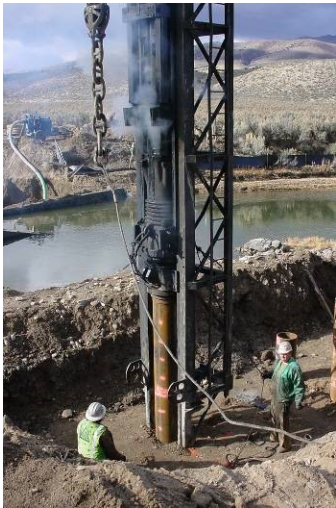
Figure 46: Pile driving operation
