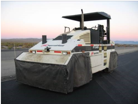
Figure 13: Rubber-tired pneumatic roller with skirting
