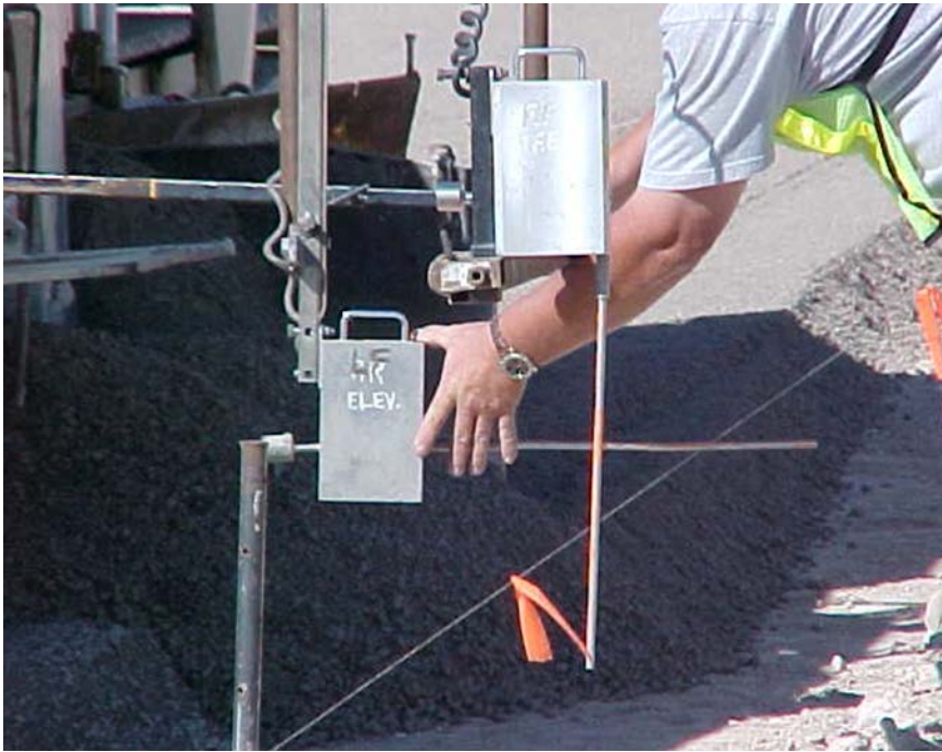
Figure 5: Setting grade controls for machine placement
