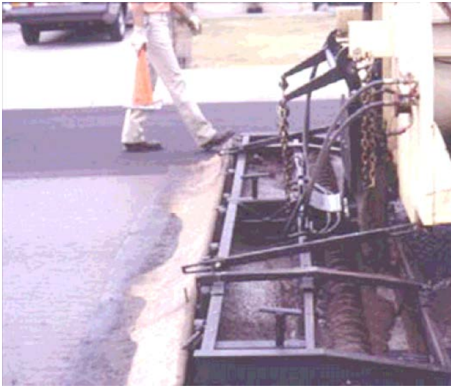
Figure 30: Spreader box and burlap
