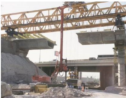
Figure 38: Segmental precast concrete box girder bridge under construction
