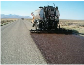
Figure 21: Distributor truck
