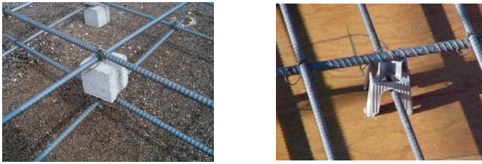
Figure 45: Typical reinforcing steel spacers and supports
