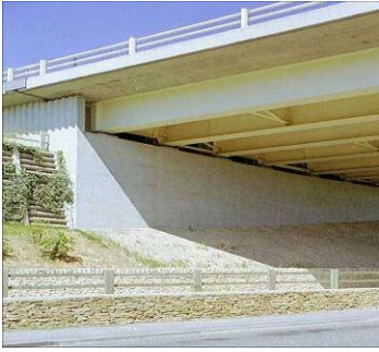
Figure 39: Structural steel bridge
