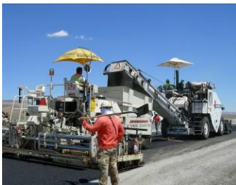
Figure 11: Plantmix paving machine
