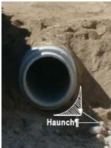
Figure 52: Pipe backfill
