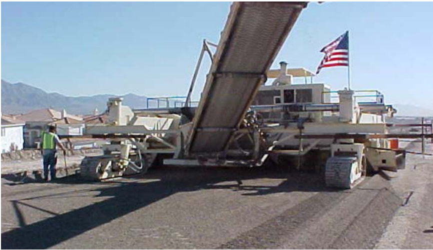
Figure 4: Class A aggregate spreader
