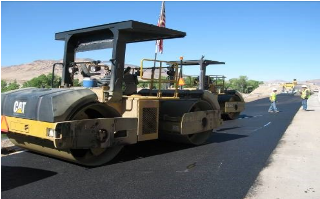
Figure 20: Double drum steel wheel vibratory roller
