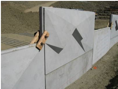
Figure 59: MSE wall facing panel
