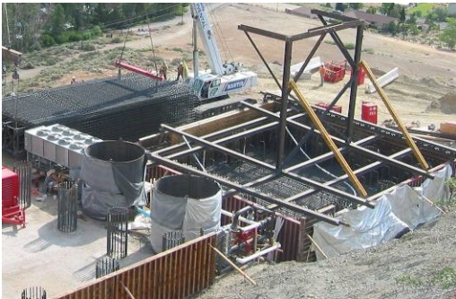
Figure 33: Cooling system for a mass concrete footing
