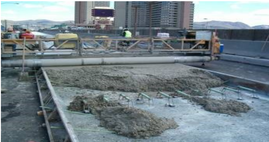
Figure 27: Side-form PCCP placement
