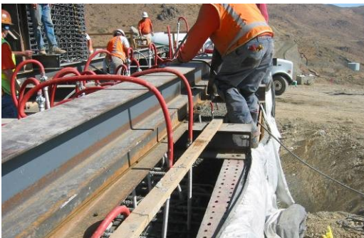
Figure 34: Component cooling pipes (red tubes) embedded in footing
