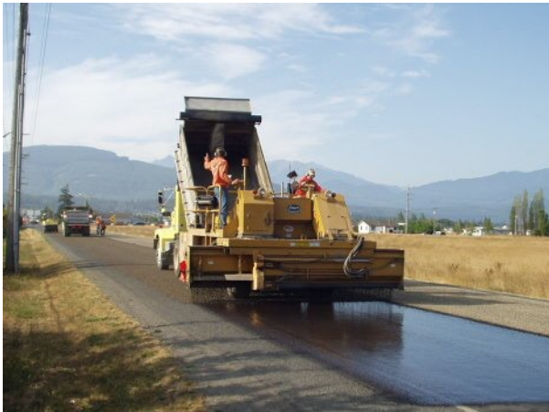
Figure 25: Chip spreader and hauling trucks
