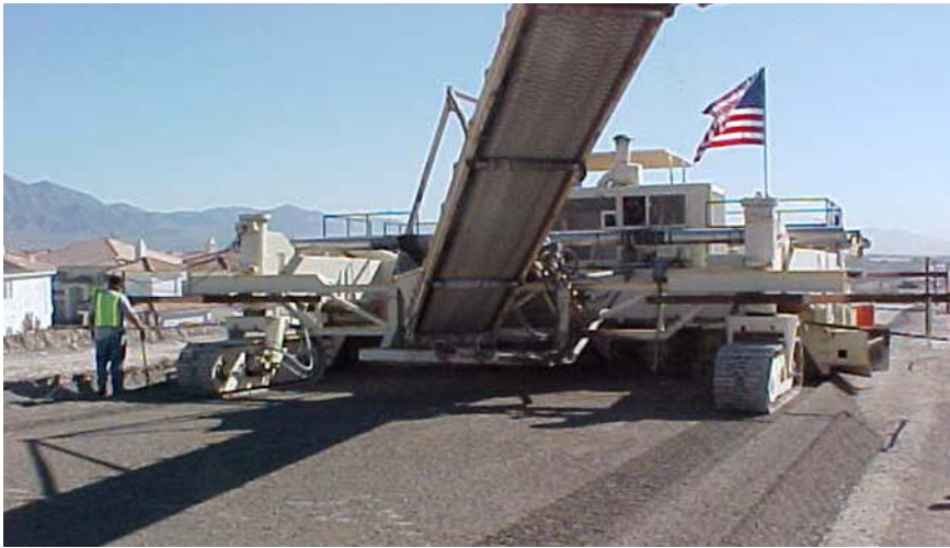
Figure 4: Class A aggregate spreader
