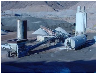
Figure 7: Aggregate marination plant
