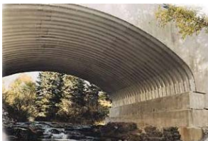
Figure 53: Structural plate culvert
