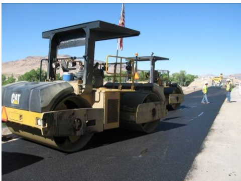
Figure 12: Steel wheel roller
