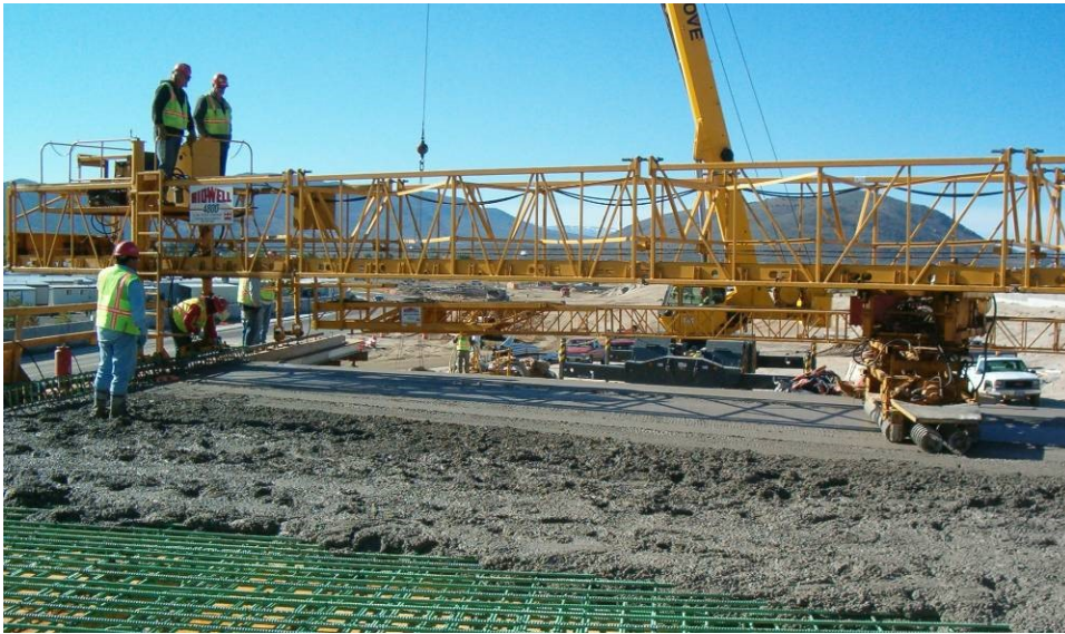
Figure 40: Bridge deck paving machine
