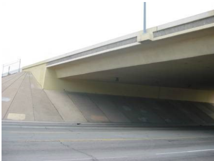
Figure 37: Cast-in-place concrete box girder bridge
