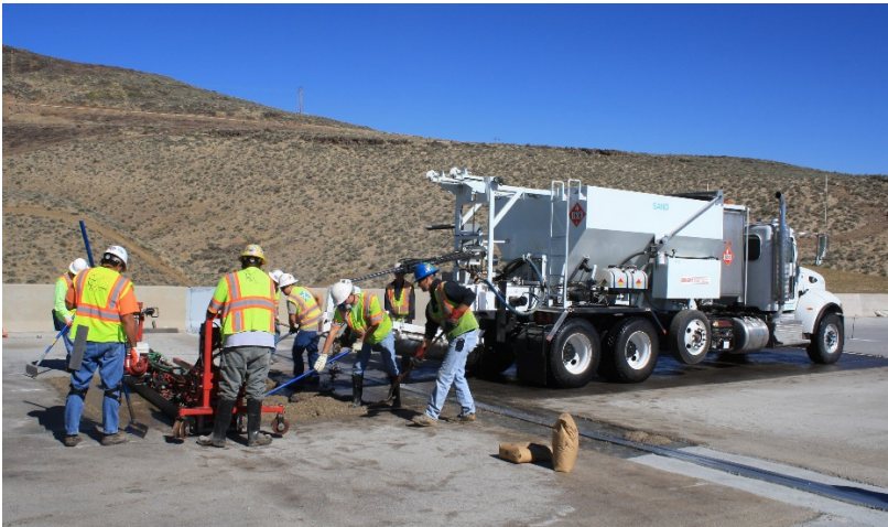
Figure 32: Volumetric mixer truck used to place polymer concrete
