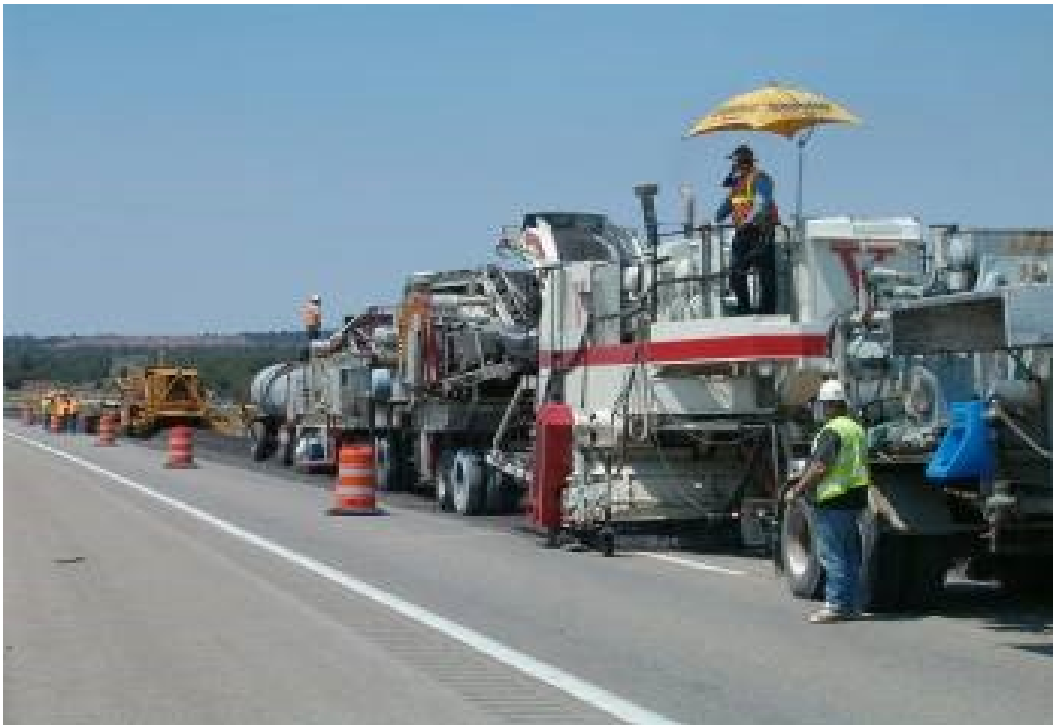
Figure 18: Recycle train
