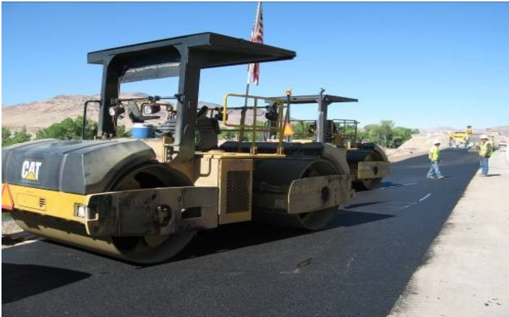
Figure 20: Double drum steel wheel vibratory roller
