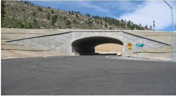
Figure 56: Typical MSE wall
