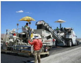
Figure 11: Plantmix paving machine
