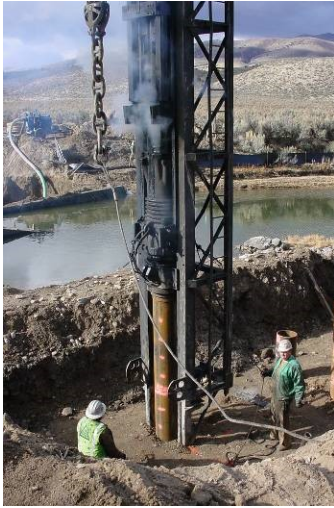
Figure 46: Pile driving operation
