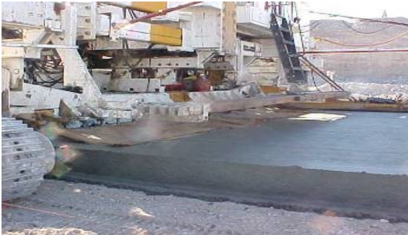
Figure 28: Slipform PCCP paver
