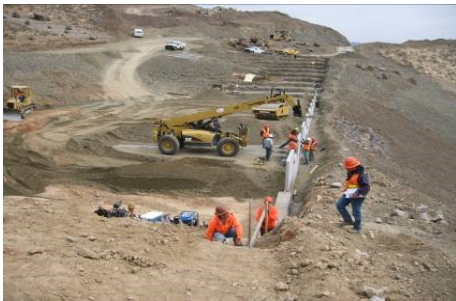
Figure 57: MSE wall installation
