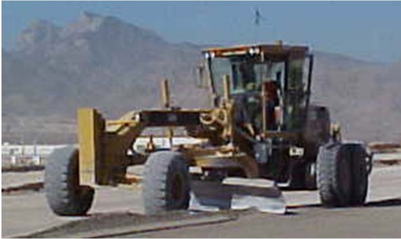
Figure 6: Windrow conditioning
