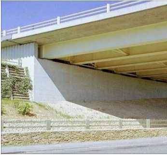
Figure 39: Structural steel bridge
