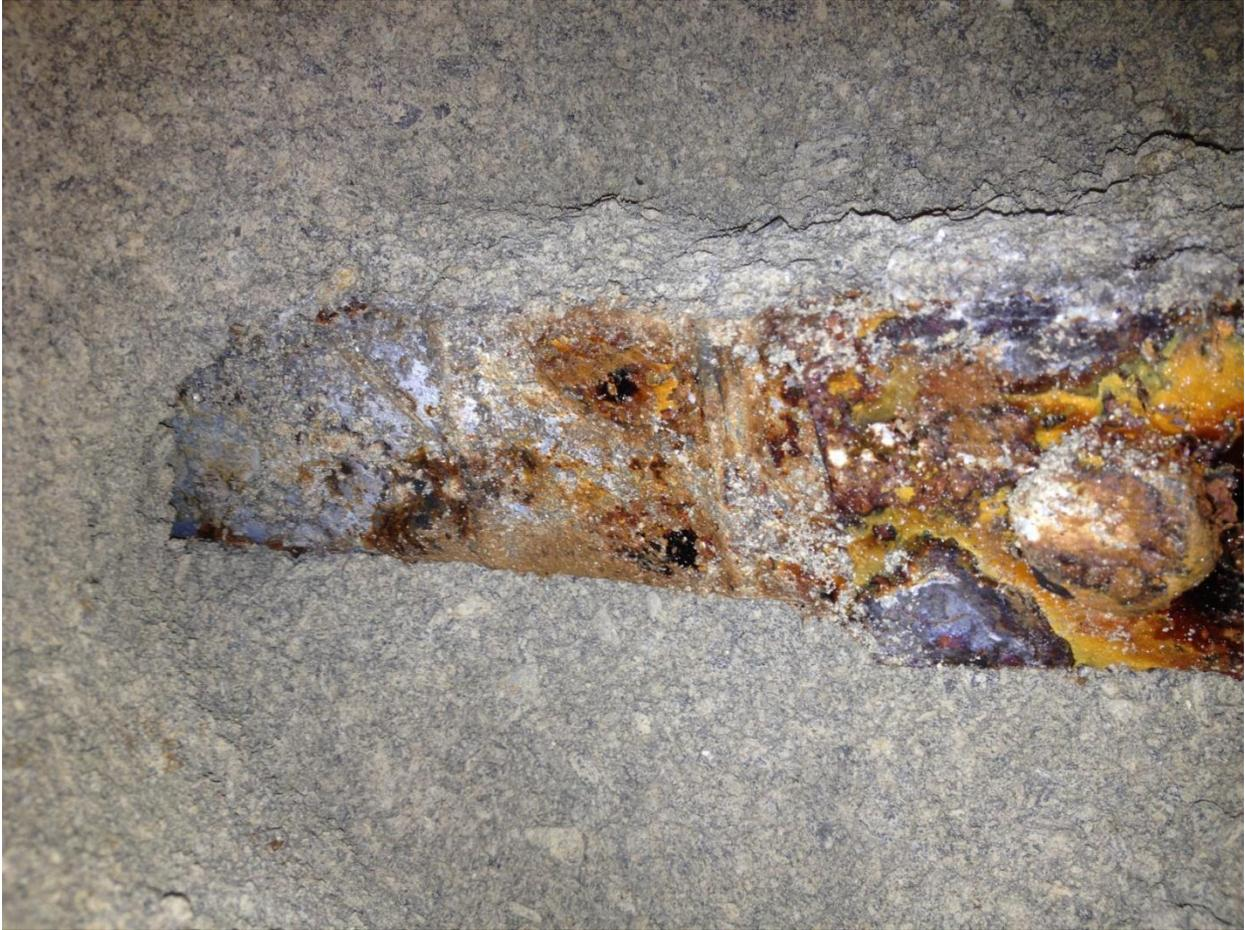
**Figure 5-13:** In-service galvanized soil reinforcement for I-15/ Cheyenne Blvd. Wall 1, 15 years old.
