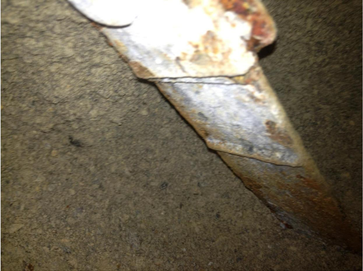
**Figure 5-12:** In-service galvanized soil reinforcement for I-15/ Cheyenne Blvd. Wall 1, 15 years old.
