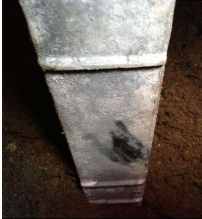
**Figure 2-2:** In-service galvanized reinforcement, a layer zinc carbonate can be seen along the surface. (ALT US 95 and ALT US 50, W1-SB-E1)
