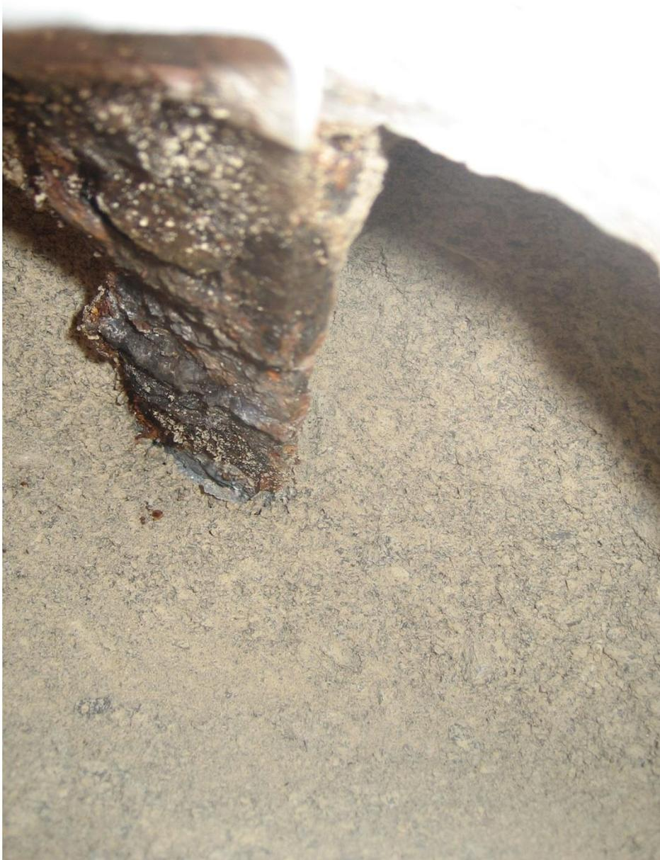
**Figure 5-15:** In-service galvanized soil reinforcement for I-15/ Cheyenne Blvd. Wall 1, 15 years old.
