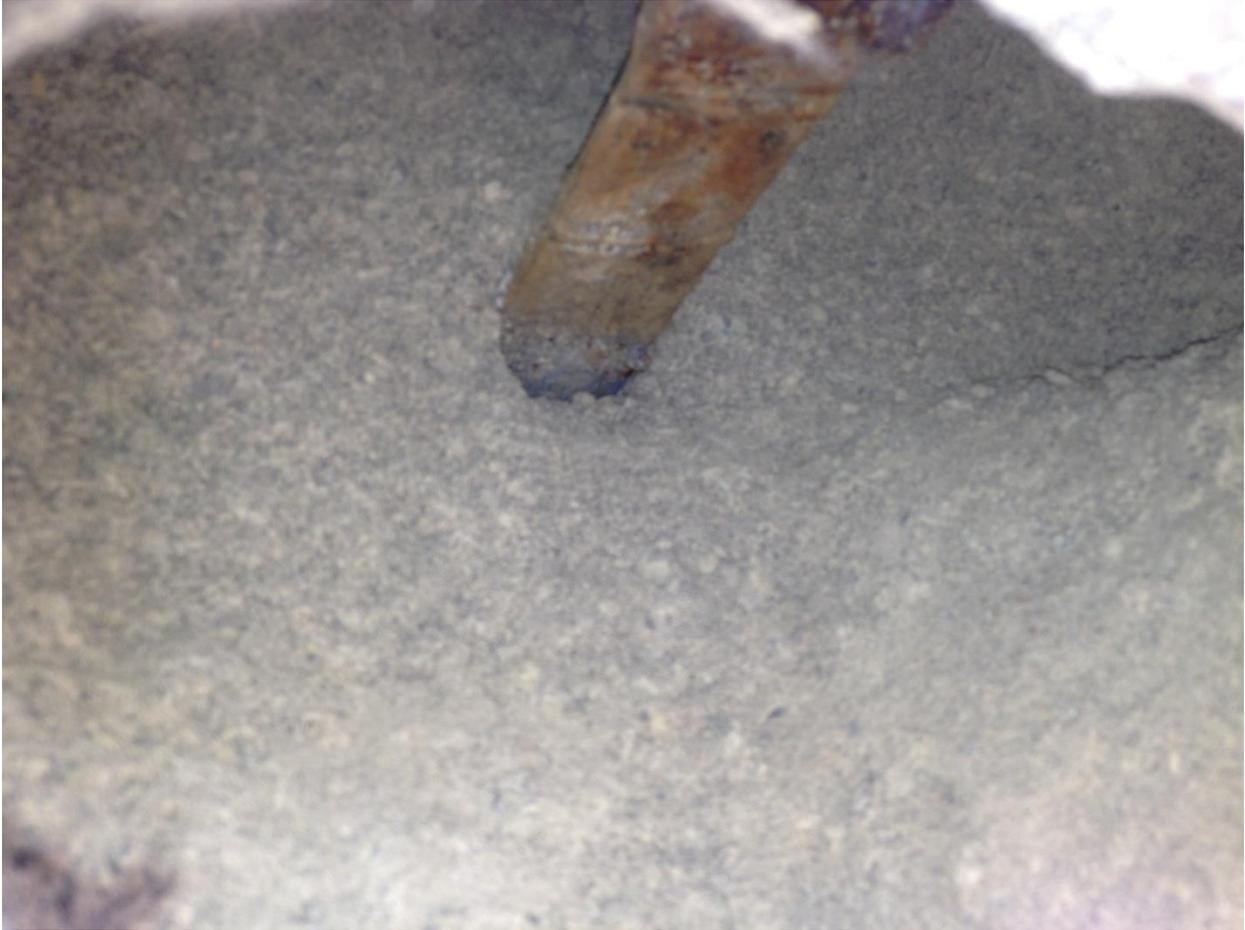
**Figure 5-17:** In-service galvanized soil reinforcement for I-15/ Cheyenne Blvd. Wall 2, 15 years old.
