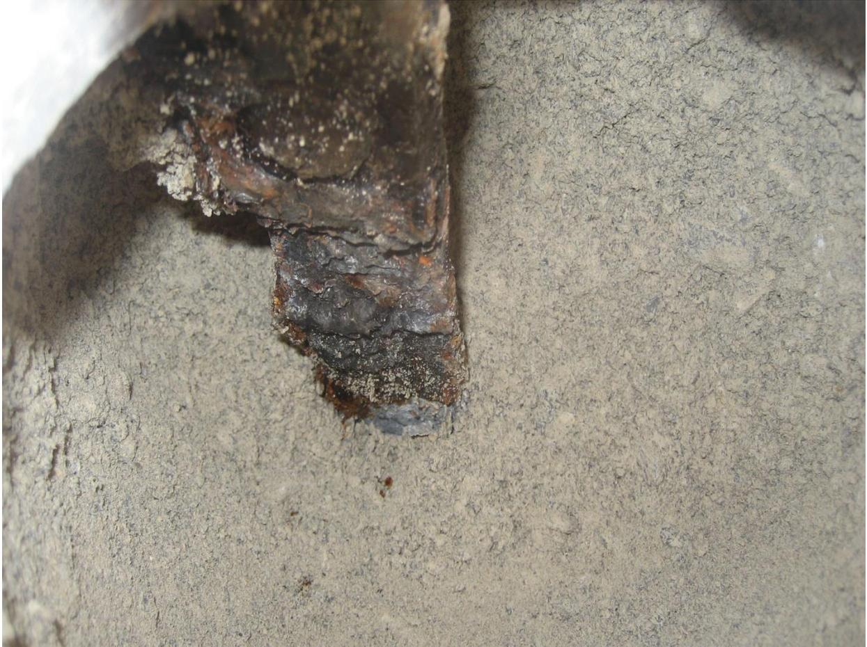
**Figure 5-14:** In-service galvanized soil reinforcement for I-15/ Cheyenne Blvd. Wall 1, 15 years old.
